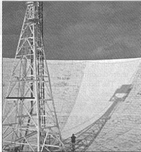
Fig 4.21: An early trial piece of the new galvanised surface. Note the thousands of mild steel plates laid during the Mk1A conversion. The ladder to gain access to the feed box is visible running up the tower. Note the size of the man standing at the base of the tower and the size of the low-loss coax cable. (Photograph by courtesy of University of Manchester Archives)
