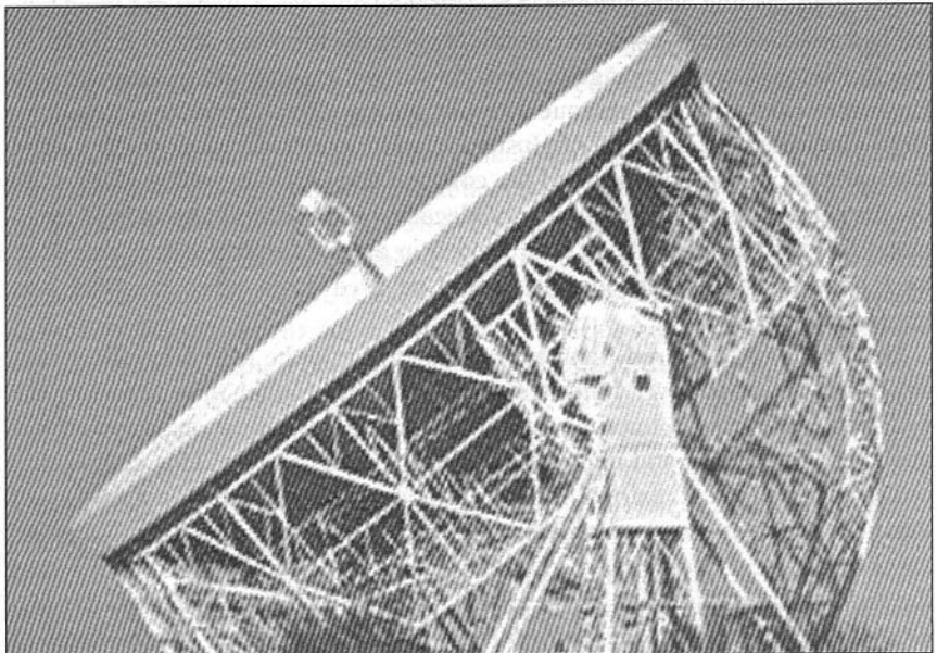
Fig 4.18: The modified Mk1A antenna shows the longer focal length and the feed box. The stabilising semi-circular twin back-girder, which replaced the original 'bicycle-wheel', was added to the back of the antenna to provide extra stiffness to the structure to relieve the stress on the elevation trunnions. The elevation trunnions are ex-Navy warship 18in gun elevation racks, salvaged from HMS Royal Sovereign and HMS Revenge when they were scrapped in 1951. (Photograph by courtesy of University of Manchester Archives)
